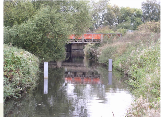
River Erewash at Attenborough showing flow meters
