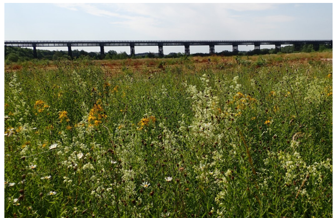
Bennerley Viaduct 25 June 2023
